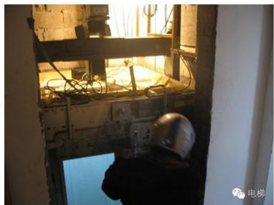
Install door operator
