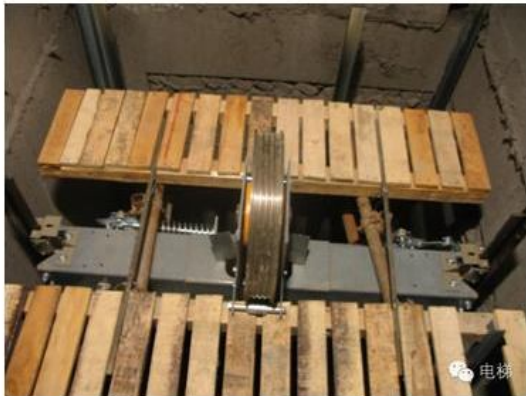
Install wood plate for temporary use, easy for shaft installation
