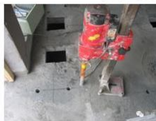
Machine room hole opening
