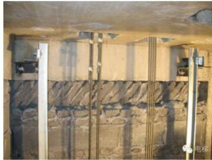
Guide rails installed
