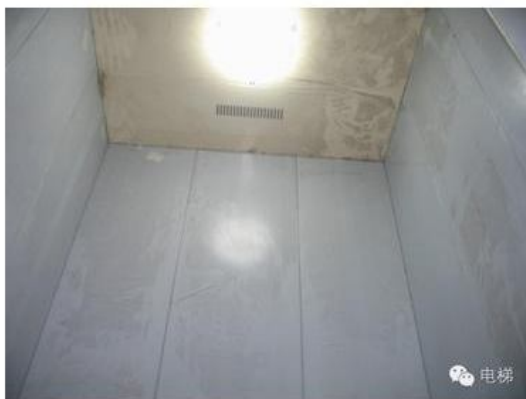
Cabin installation finish
