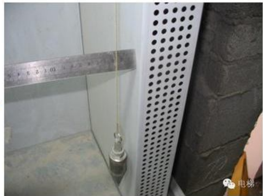
Adjust cabin and finish cabin fixing
