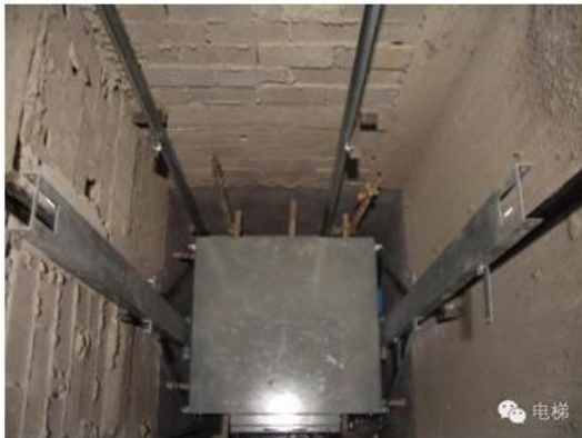
Install cabin flooring
