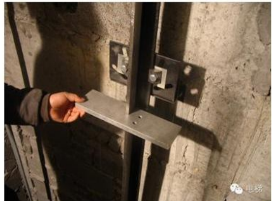
Fixing brackets ( with self-made ruler)
