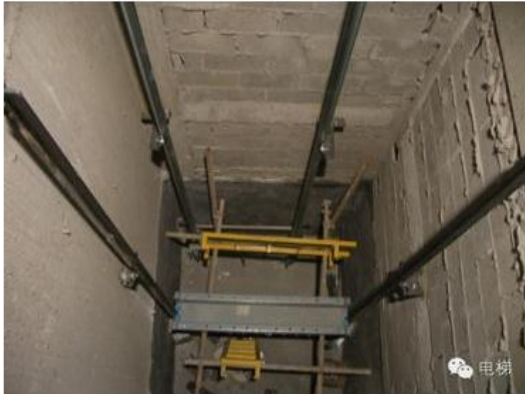
Install bottom beam after one piece of guide rail installed
