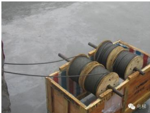
Install steel rope
