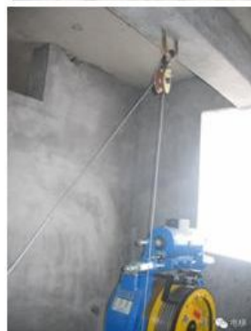
Fix hoisting machine for guide rails lifting/installation purpose
