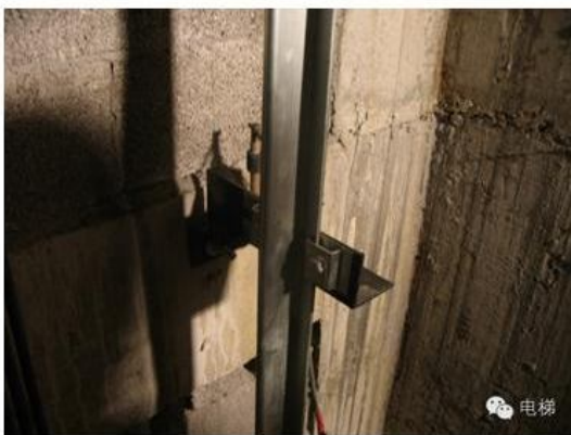
Fixing CW rail brackets
