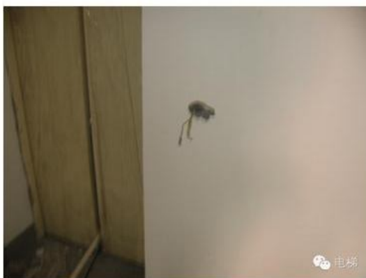
Boxless HOP cable hole
