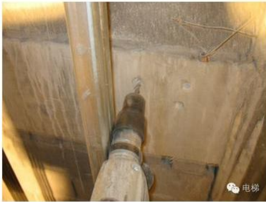
Drilling hole for CW rails
