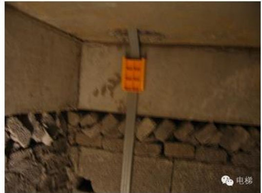
Fixing travelling cable on top of shaft
