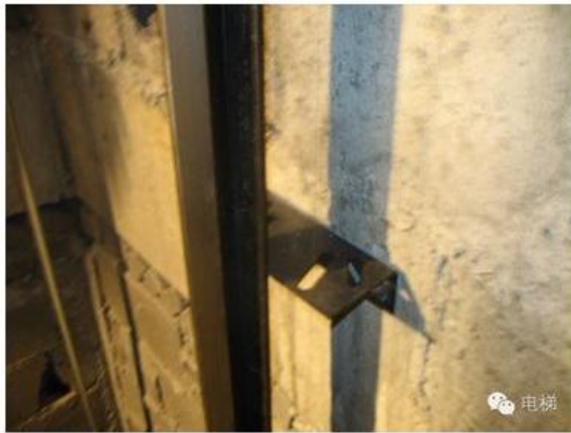
Fixing rail supports
