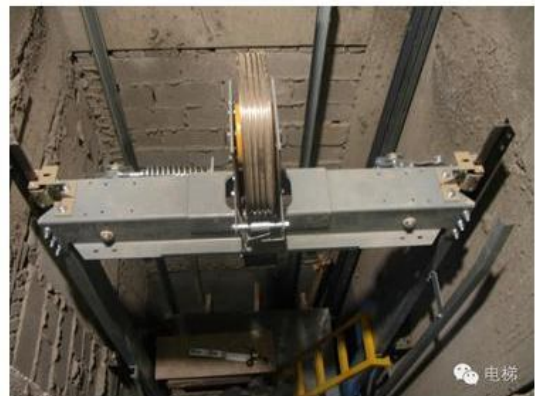
Install up beam and sheave
