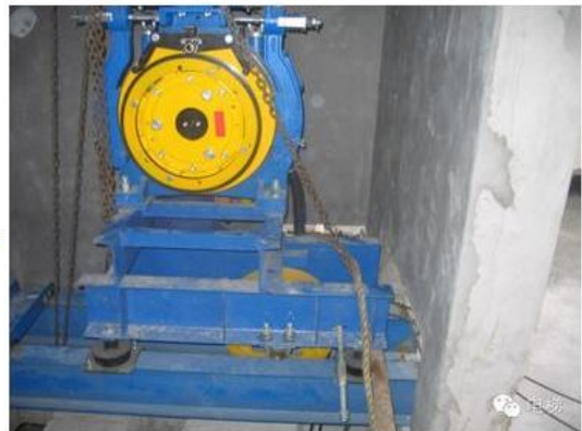
Hoisting CW frame
