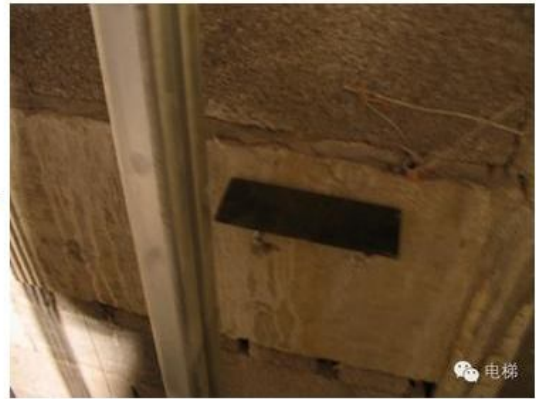
Fix CW rail support
