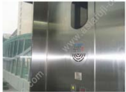
Luo maicao-based near the east arch liaison office flyover of escalators
